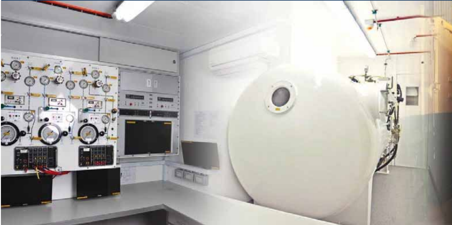
Dive Control Container
